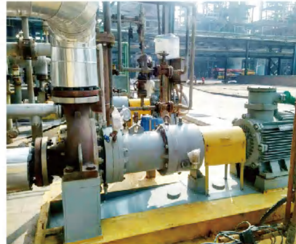
多晶硅 急冷塔循环泵 Rapid cooling tower circulating pump for Polycrystalline Silicon 流量Q : 150m 3 /h 扬程H : 53m
