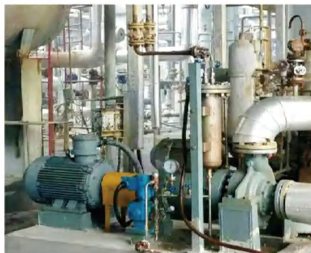
泥浆型磁力泵 含固料50% Slurry magnet pump, transferring material with 50% solid particle 流量Q=160m 3 /h 扬程H=95m
